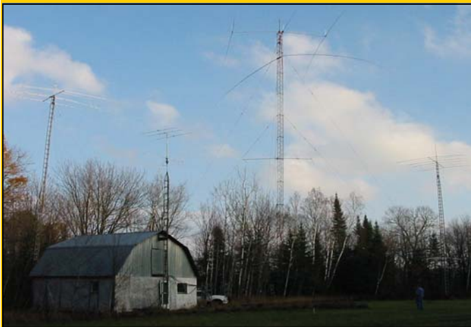
The antenna farm at VA3SK's in North Bay includes (from left to right) a High-gain Explorer with 40 meter extensions at 56'; a six meter beam affixed to the operating stable (it's a long story); the homemade full-size 3-element 40 meter beam at 110' with an 80 meter single-element dipole and 15-meter beam fixed on Europe; finally a TH-7 at 56' with another 15-meter fixed beam.
