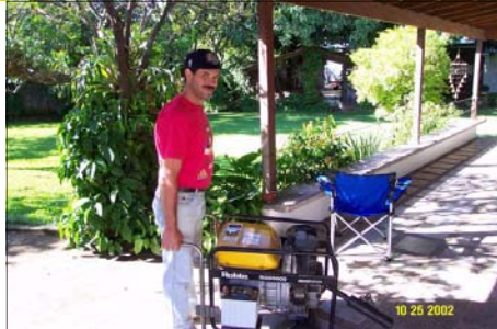
Standby Generator that didn't quite make it!!
